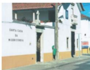
Fachada Principal SCMA
